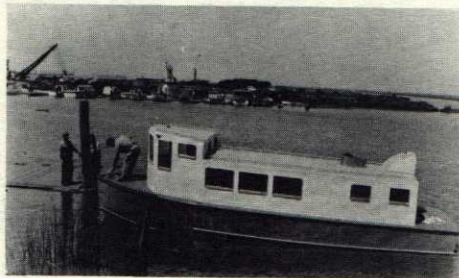
River Launch work, N. Peru
