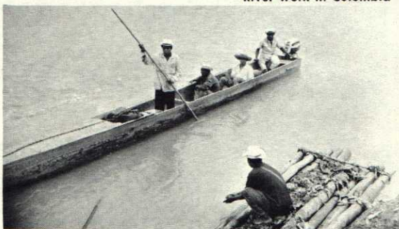
River work in Colombia
