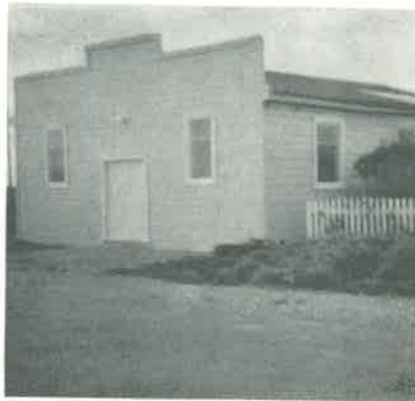
Gospel Hall, Tokomaru, opened September, 1956, where the assembly now meets.
