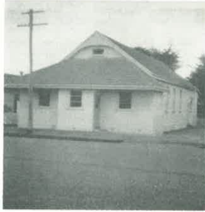
Gospel Hall, Oxford Street, Levin, 1956, after alterations had been effected.
