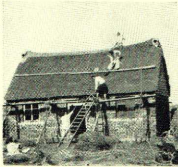
The final mud plaster being put on a newly thatched roof
