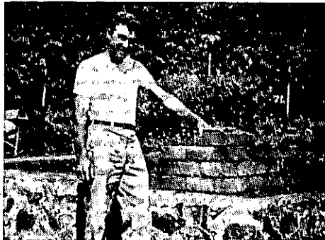
Robert Milburn constructing at Nyankunde
