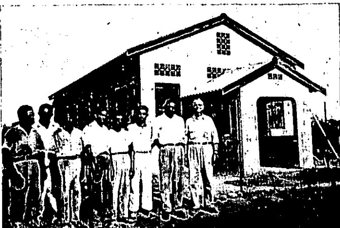
Mr. Williams and his helpers outside the new Sorpresa Hall.
