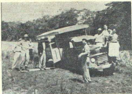
Hazardous Road in Paraguay
