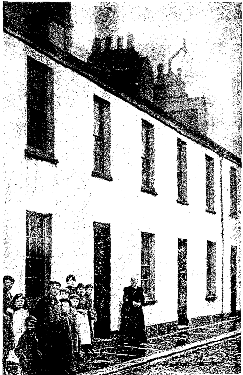
THE HOME OF R. C. CHAPMAN, No. 9, New Buildings, Barnstaple.
