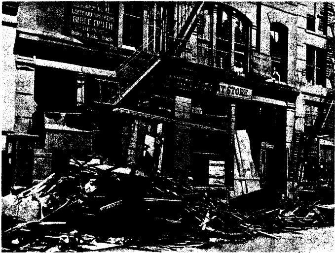
This Sight Greeted the Staff on Monday, April 21, 1919, After the Fire at 1 East 13th Street
